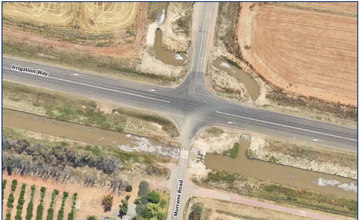
Figure 2.12: Irrigation Way and Murrami Road Intersection
