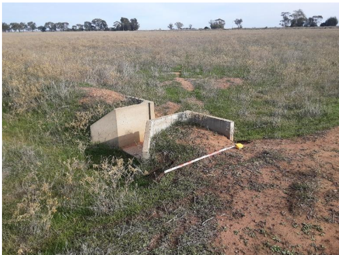
Photo 10 Area of higher visibility (20%) within the east of the study area, photo facing south showing drainage infrastructure
