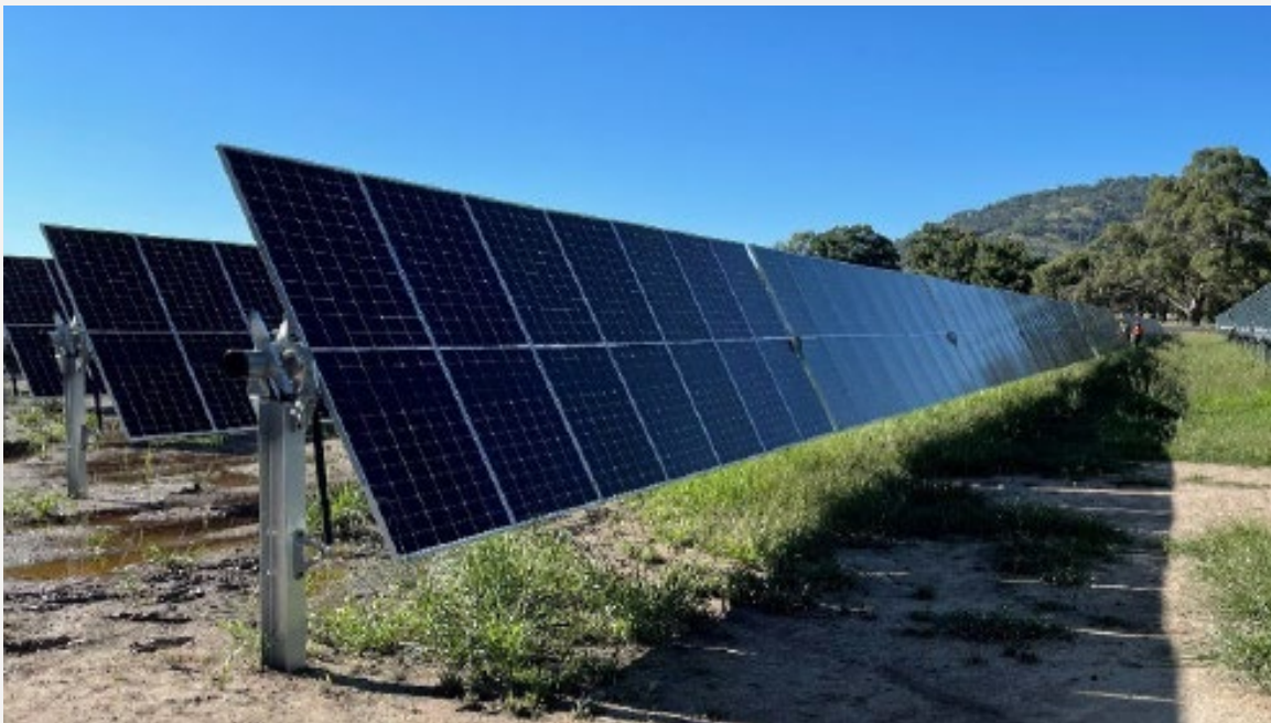
Figure 9 | Example of a Typical Single Axis Tracker System with PV Modules Mounted in Single Panel Portrait Orientation (1P Configuration)
